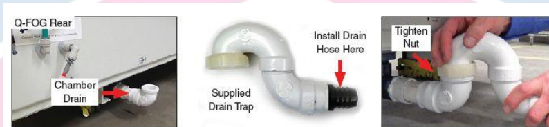
Figure 6.6a: Drain trap installation.
