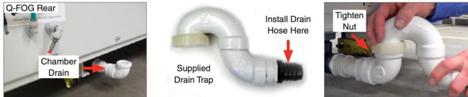
Figure 5.8a: Drain trap installation.
