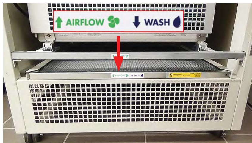
Figure 15.5.d: Make Sure the AIRFLOW Arrow Points Up
