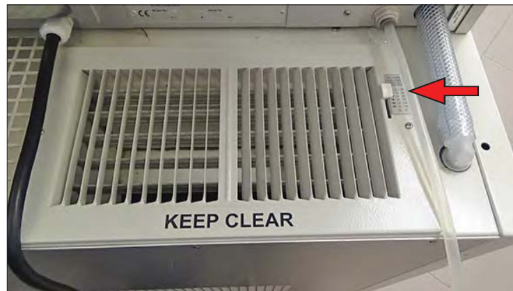
Figure 11.2d: Xe-1-BCE and Xe-1-SCE damper adjustment.
