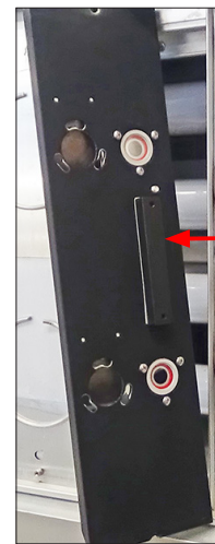
Figure 8.1b: Interior of black panel showing uninsulated temperature sensor.
