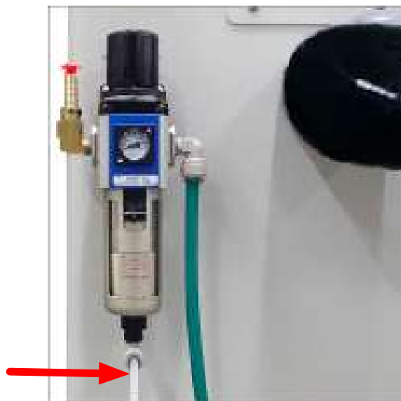
Figure 6.6g: Air filter drain location.
